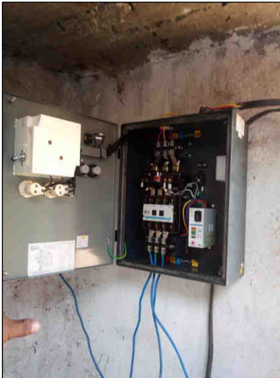
Repairing of Panel and wire Submersible Pump (3HP) at Near Panjab National Bank ward No 10 Nariyara
