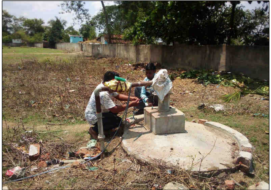
Repairing Panel and wire of Submersible Pump (5HP) at Bastipara OHWT Rogda
