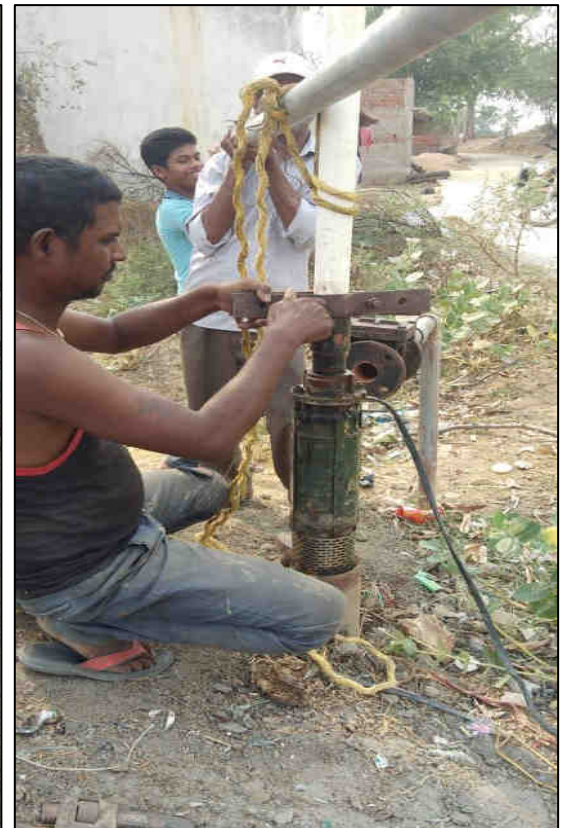
Shifting and Installation of Submersible pump (3HP) word no 18 Near Mukti Dham Nariyara
