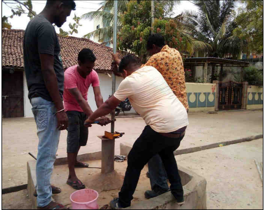
Repairing of Handpump ward No 02 Nariyara village
