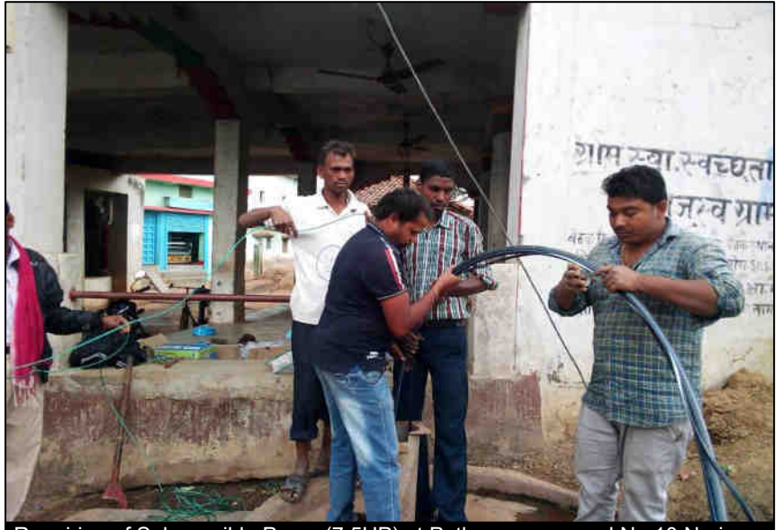
Repairing of Submersible Pump (7.5HP) at Patharra para ward No 10 Nariyara
