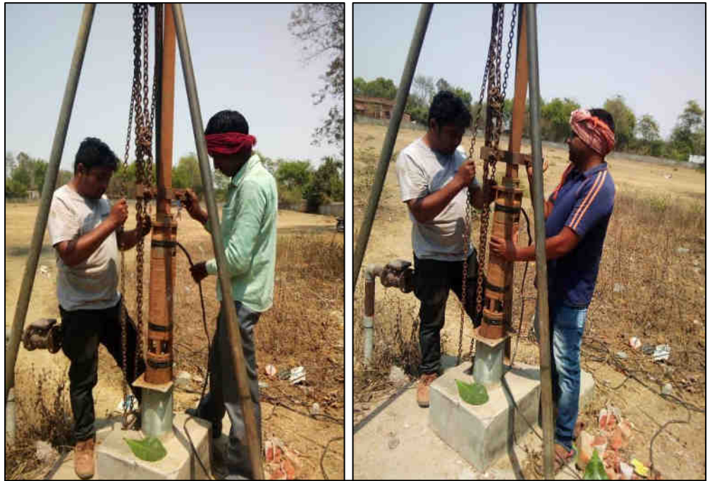
Repairing of Submersible Pump (5HP) at OHWT Rogda
