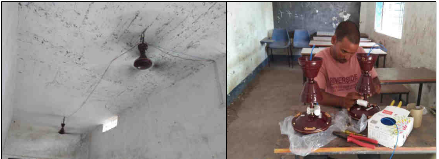
Fitting of 04 Nos ceiling Fan and Electrification at Govt. Middle School Rogda Village
