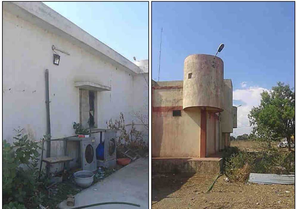
Installation and repairing work of 6 Nos Street light at Police Station Mulmulla
