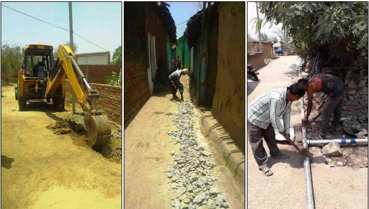
Pipeline Extension work 300 meter ward no. 6, 13, and 16 at Nariyara village
